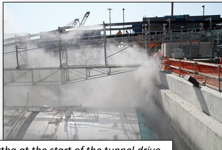
Bertha at the start of the tunnel drive.
