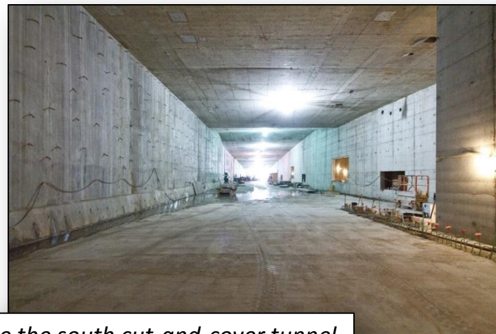
Inside the south cut-and-cover tunnel
