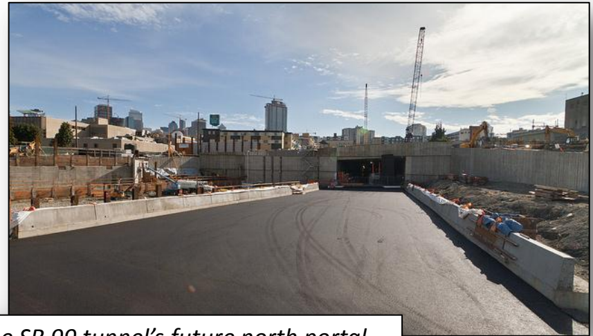
The SR 99 tunnel's future north portal.
