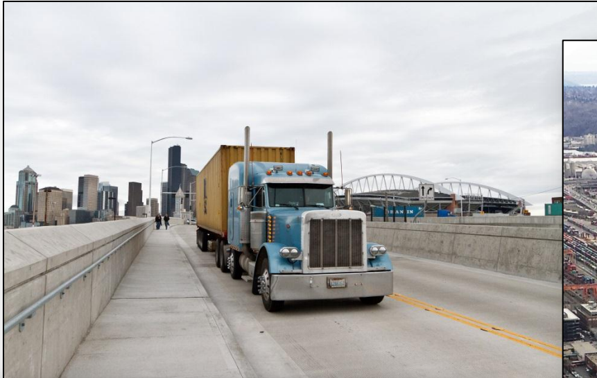
Holgate to King: the South Atlantic Street overpass
