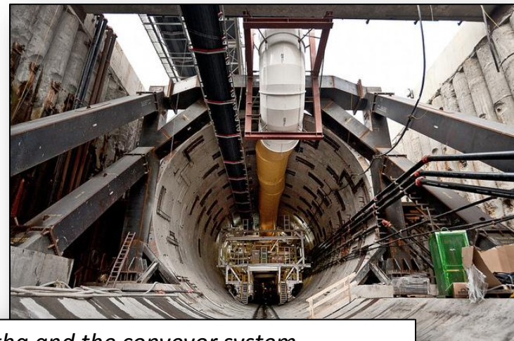
Bertha and the conveyor system.
